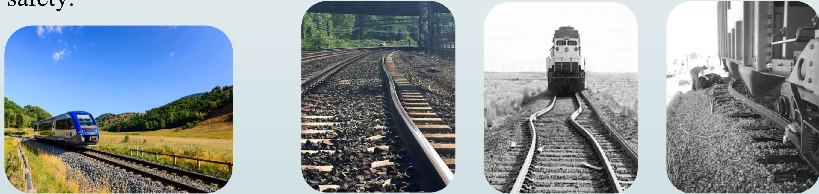
Exploitation → Geometrical defects
