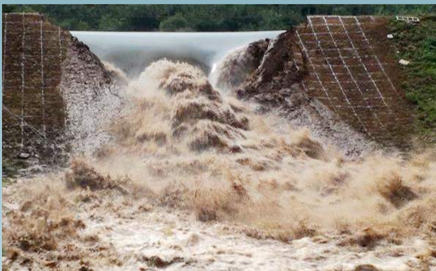
Figure 1: Dam failures caused by internal erosion
